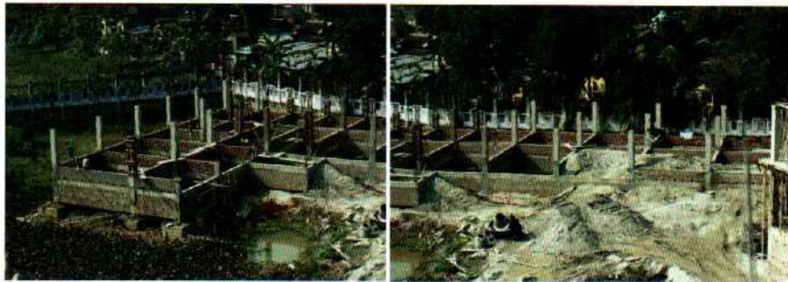
A VIEW OF UNDER CONSTRUCTION SEMINAR HALL (W.I.P. 25%)
