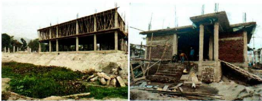
A VIEW OF UNDER CONSTRUCTION EVALUATION HALL (W.I.P. 50%) EMERGENCY BLOCK (W.I.P. 85%)
