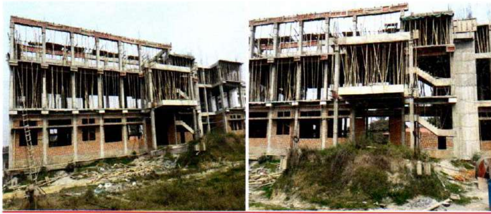
A VIEW OF UNDER CONSTRUCTION OF ACADEMIC BUILDING
